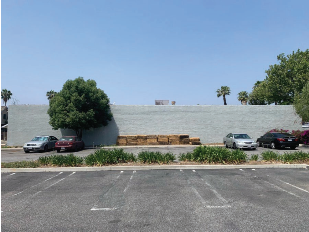
EAST SIDE OF UNIT FROM ADJACENT SITE
