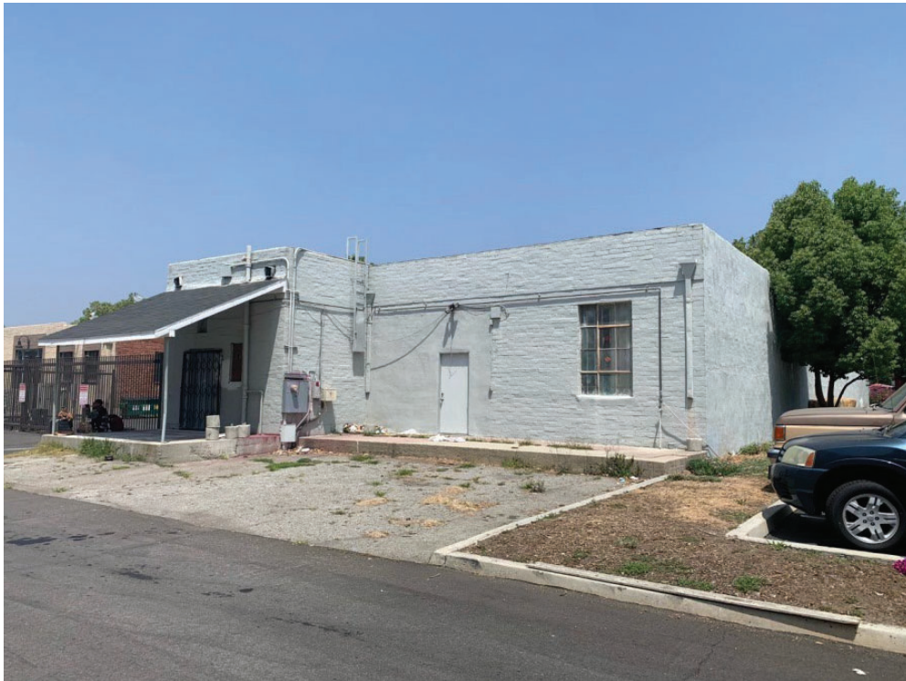
REAR OF UNIT
