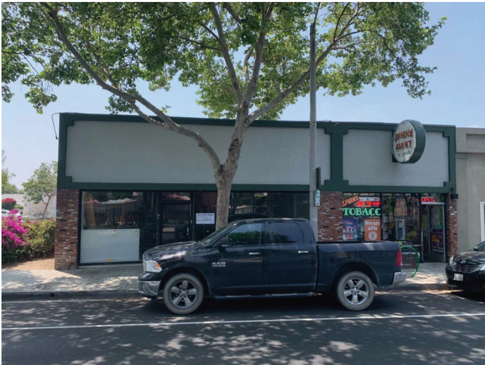
FRONT OF UNIT FROM STREET
